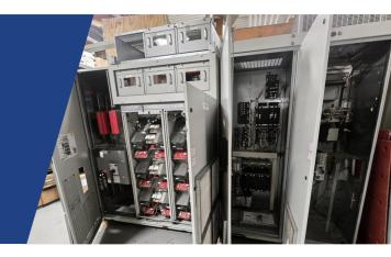
EX2100™ exciter bridge fans installed between approximately 2000 and 2008 are beyond or near the end of their designed life, increasing the risk of failure. These fans are critical to safe and reliable AVR operation, with an OEM recommendation to replace them every four years or less.
